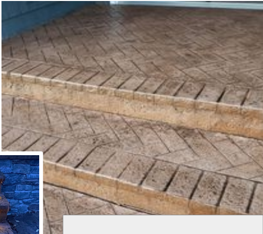
Cantilever style (integrated lip) steps with traction strip inserts. These strips are an important consideration when there is no plan to install a handrail.
