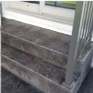
Flat faces and flat sides with lightly stamped treads
