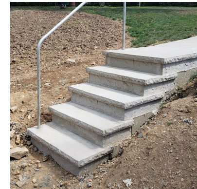
Cantilever style (integrated lip) steps in plain concrete with brushed treads
