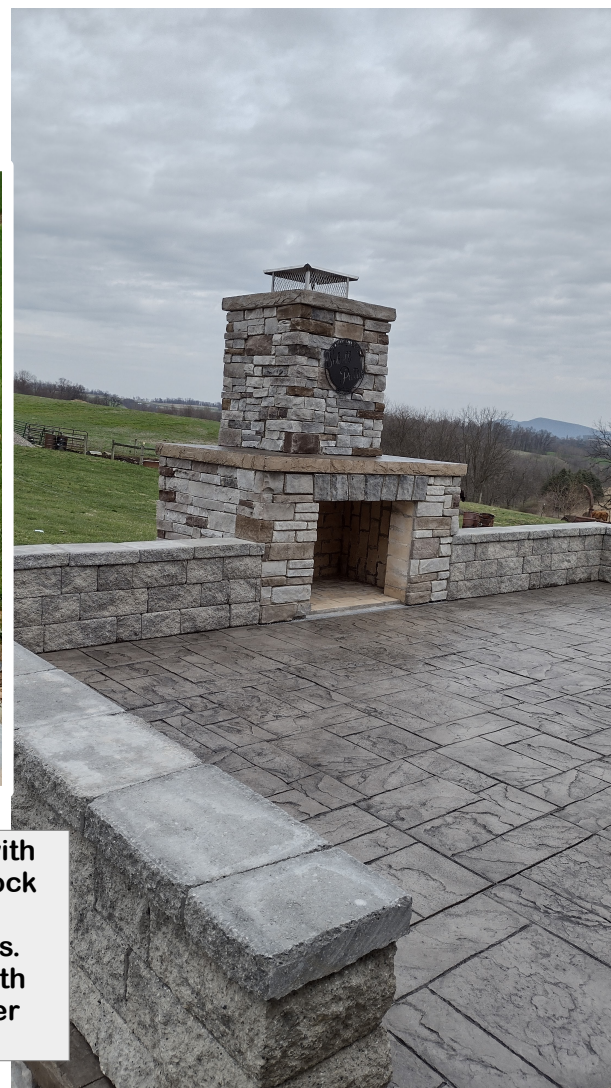
A bi-level Weatherwood Plank patio with a built in grill, pot heater, and propane fireplace. Double access doors and storage drawers are built in. The step at the door is a matching wood plank cantilever style step. The stone veneer is Dutch Quality and the wall caps are paver style caps. All propane and electrical lines are buried in conduit under the concrete slab. The picture below shows the process of building the kitchen to fit the chosen appliances.
