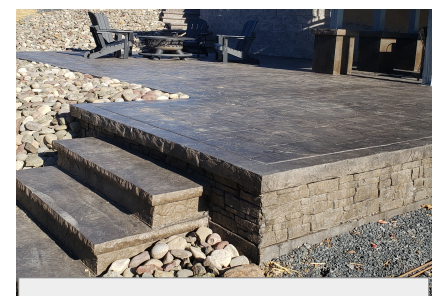
Patios with raised sides can be placed as monolithic slabs with liners used to texture the exposed concrete instead of plain flat walls. This works well when the sides are 16 – 18" high.
