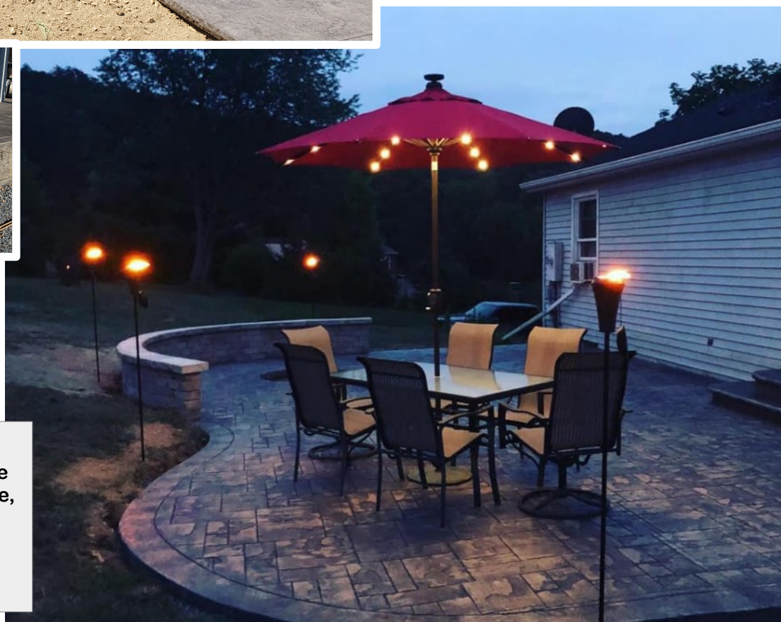
Patios with raised sides can be placed as monolithic slabs with liners used to texture the exposed concrete instead of plain flat walls. This works well when the sides are 16 – 18" high.
